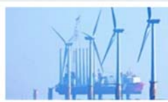
Green Energy Rush Hit by Headwinds
